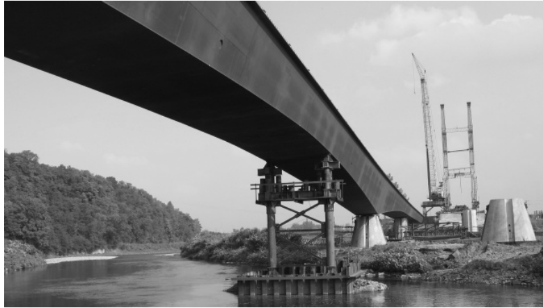
Steel-concrete composite bridge on highway D47 under construction from weathering steel
