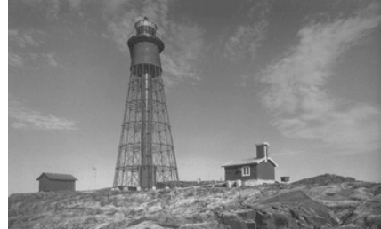
The lighthouse Pater Noster is one of the first duplex treated steel constructions in Sweden. It was galvanized in 1868, and after that painted
