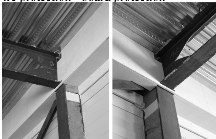
Board fire protection at fire test in Mokrsko, 18 September 2008
