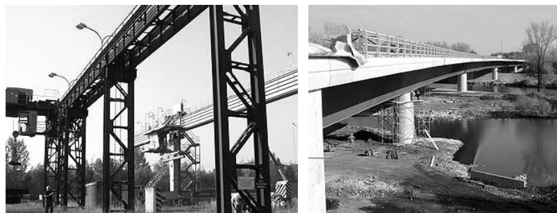
Example of structures from weathering steel
